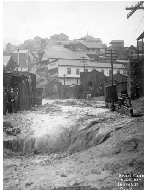
This 1903 Bisbee (Ariz.) flood destroyed many homes and businesses. While floods continue to haunt the state, they were worse during Territorial days. Arizona State Archives #96-3378. Humphries Photo.
