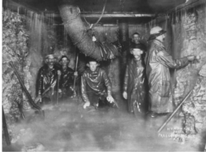
In the late 1800s and early 1900s, the mines in the town of Tombstone were subject to increased flooding. Despite massive efforts to pump the water out, mining eventually had to be abandoned. Today, some Tombstone streets are collapsing into these abandoned shafts. Humphries Photo. Arizona State Archives #97-0429.
